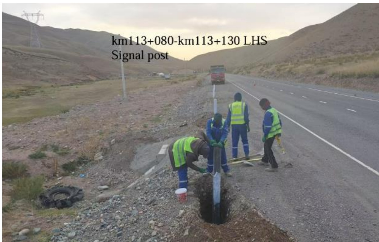
Рисунок 12: Signal post installation, km113+080 - km113+130 LHS
